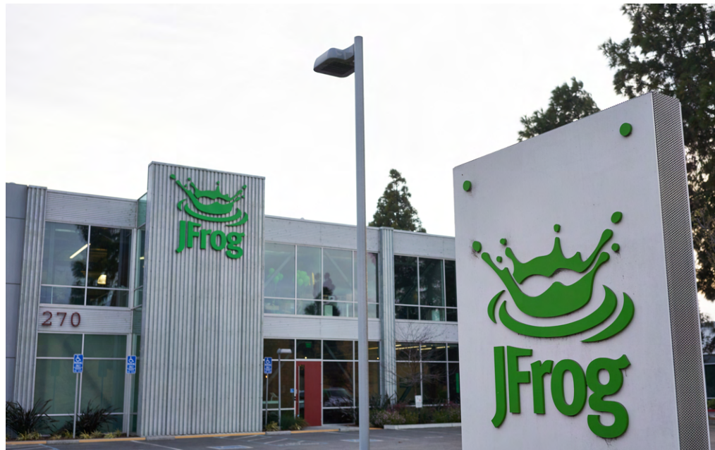
JFrog's green building in Sunnyvale, CA
